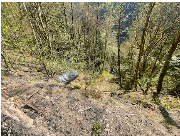
Downslope and culvert.
